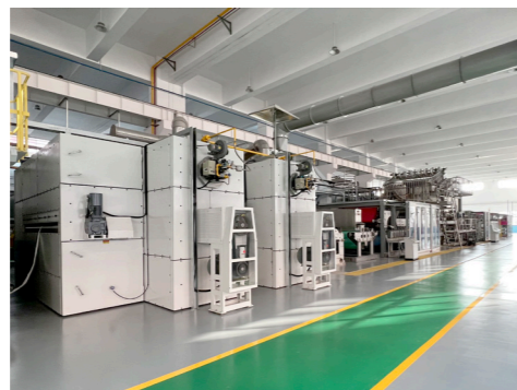
飞龙生产线 Production line of Feilong
